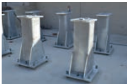
Fixing of Base Plates
