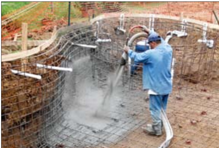
A builder sprays gunite to create a suburban pool
